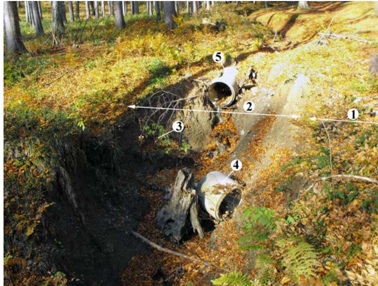
Figure 12. The channel of the Bozsoki Valley at profile marked I. (time of picture 30.10.2010) Legend: floor of Bozsoki Valley, 2. channel, 3. collapsed part of channel side, 4. moved bridge part (concrete ring), 5. concrete ring of the bridge which is stable.
