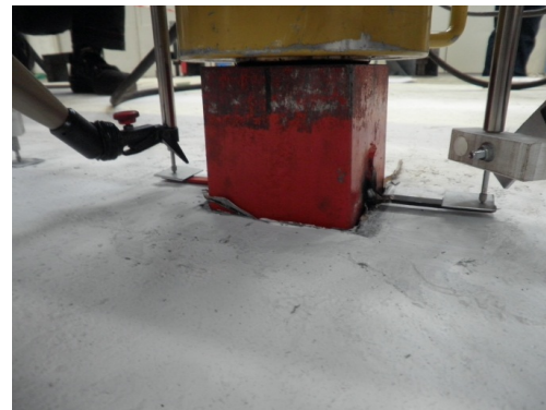
Figure 8. Crack patterns and failure for centre load [15].
