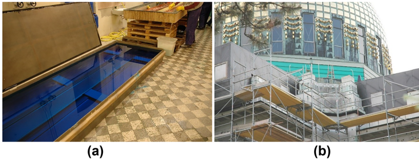
Figure 1: Artificial brochantite patination for the tambour sheeting of the Otto Wagner Church in Steinhof, Vienna, 2004. (a) Bath with submersed copper sheet, (b) tambour with new sheeting. © University of Applied Arts Vienna.
