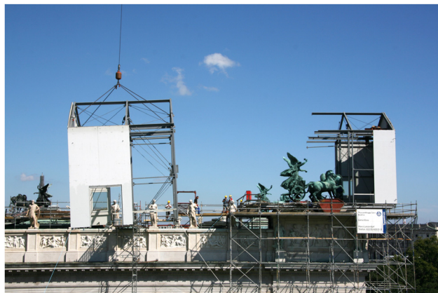
Figure 7: Construction of the housing on the roof of the Austrian parliament for the restoration of one of the Quadrigas. © Parlamentsdirektion, Michael Buchner, Picture ID: 2652377. Date of photograph: 22.08.2007.
