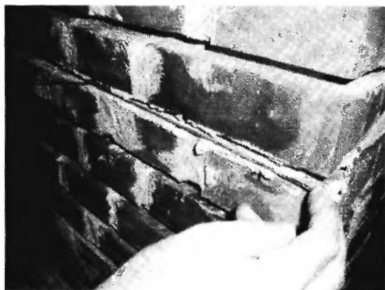
Fig. 1: Placement of the strip and repointing with mortar.
