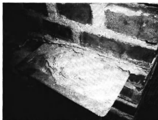
Fig. 1: Placement of the strip and repointing with mortar.
