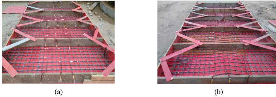
Figure 4: The formwork of one-way concrete slab specimens. (a) Distribution of straight steel bars and (b) distribution of SCAHSs.
