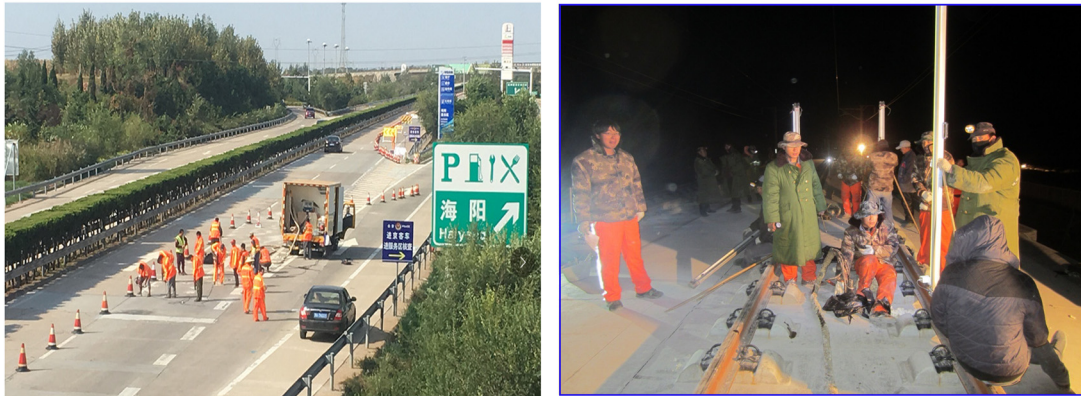
Figure 1: Engineering application of nonwater reacted polyurethane grouting materials.
