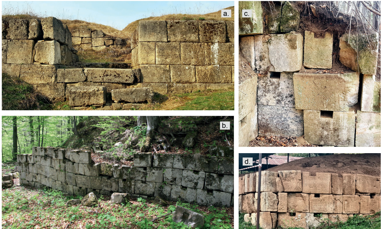
Fig. 3: Ashlar masonry at the Dacian fortresses in the Șureanu Mountains: (a) The entrance to the Dacian fortress at Costești-Blidaru; (b) Retaining wall at Sarmizegetusa Regia; (c) Retaining wall at Fețele Albe; (d) Residential tower at Costești-Cetățuie.
