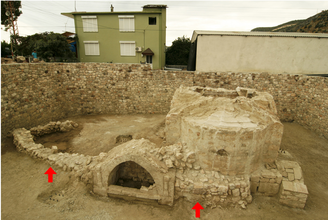
Figure 1: The church and tombs in Myra, view from the east. Red arrows show the protective wall constructed against flood water (Myra/Andriake excavation®).
