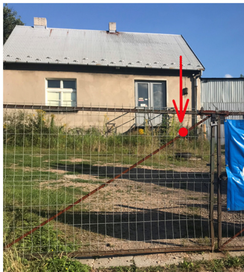
Figure 10: Photograph of building with inaccessible point.
