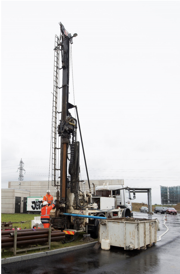
Figure 2: Core drilling. Photo: Per Lindh.
