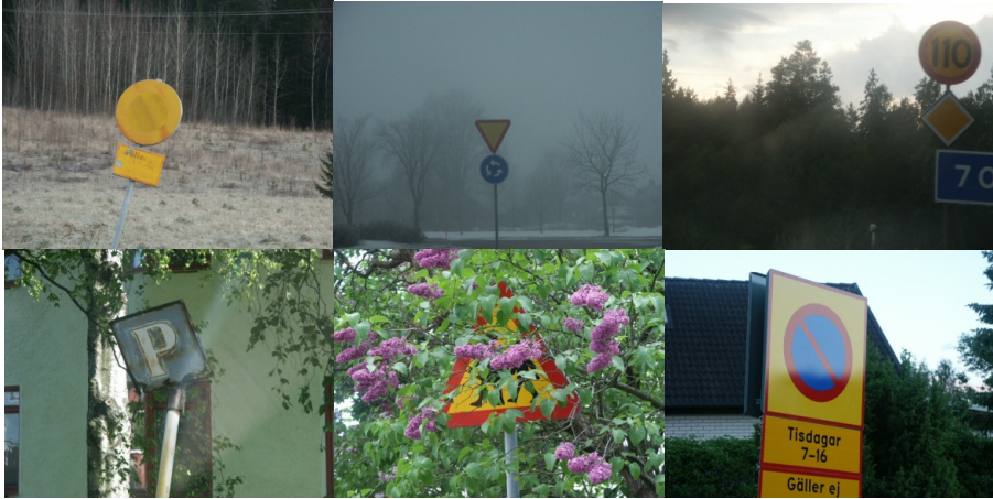
Figure 1. Potential difficulties when dealing with signs, from upper left to bottom right: Faded, Challenging weather conditions, Bad lighting geometry, Damaged sign, Occluded sign, and Highlighted sign.
