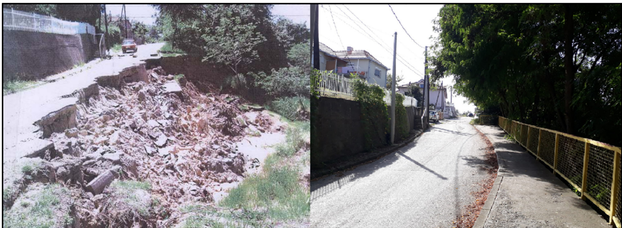
Figure 3: Dunavska Street: during the landslide (2007) – left, and landslide recovery (2023) – right.
