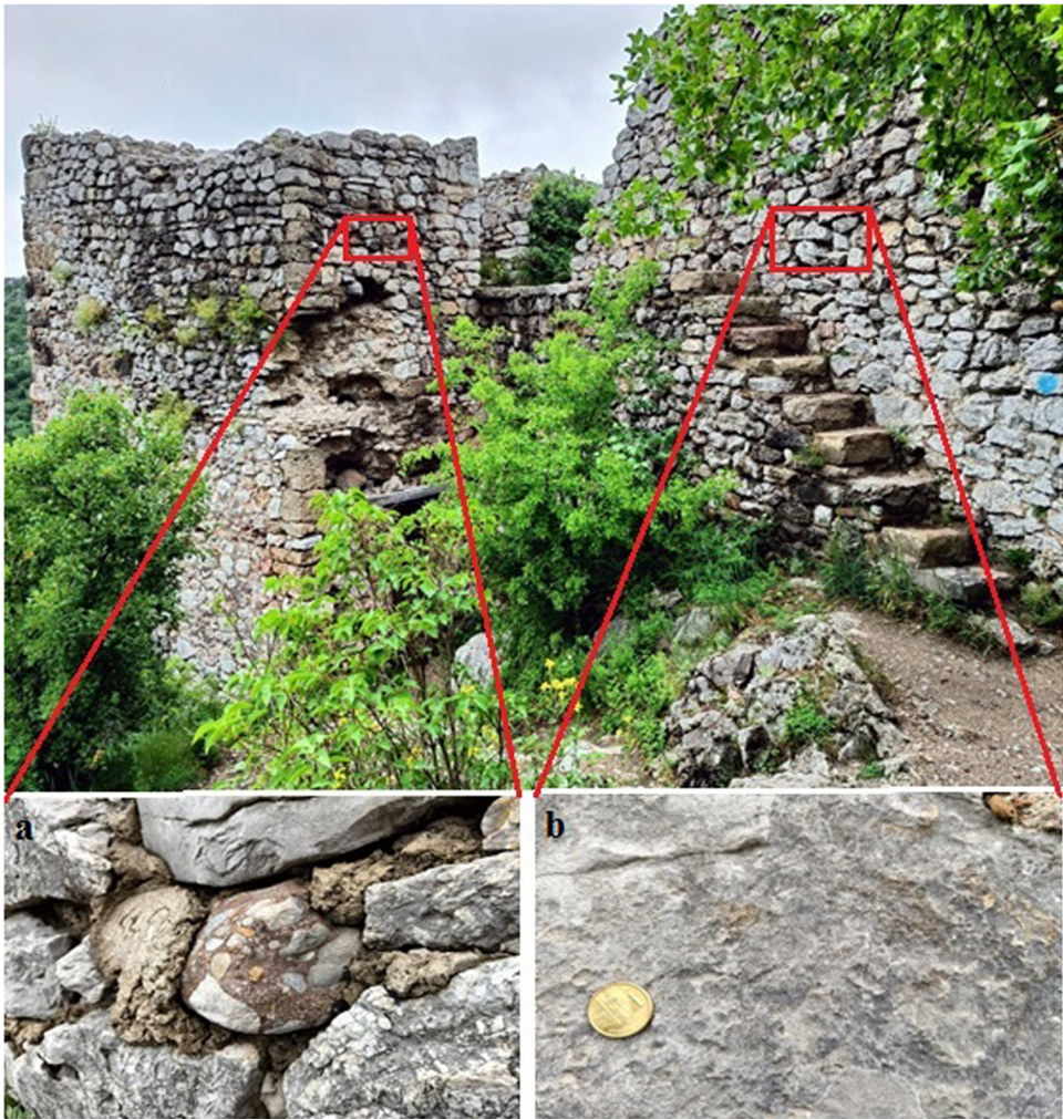
Figure 5: Main building stone visible on the site: (a) conglomerates built in the entrance gate and (b) limestone blocks used for the defensive walls.
