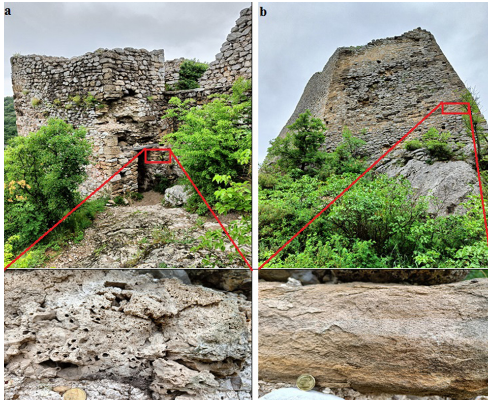
Figure 6: Building stone material used for the entrance gate: (a) tufa blocs with visible macro-biological components and (b) sandstone blocks used for the defensive tower.
