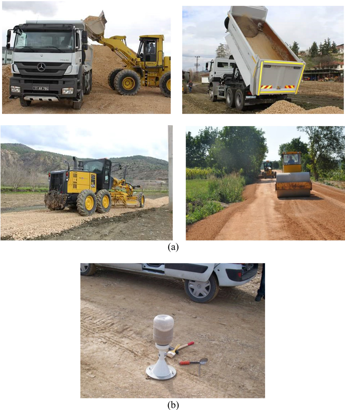
Figure 10: (a) Compaction of the base layer made of marble waste and (b) control by sand cone method on the base layer.
