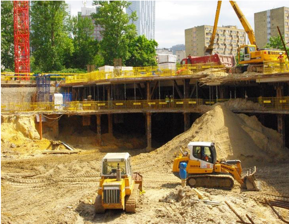
Figure 1: Excavation supported with a top-down method (photograph by Janina Zaczek-Peplinska).
