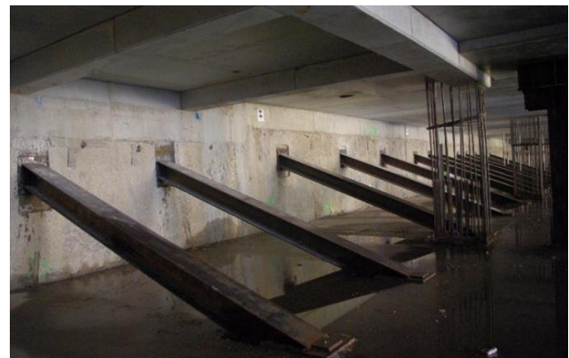
Figure 3: View of the diaphragm wall at level -1 (-4.70 m) (photograph by Janina Zaczek-Peplinska).
