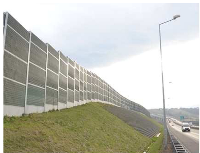
Figure 8: Overview of the slope with retaining structure and the noise barriers [33].
