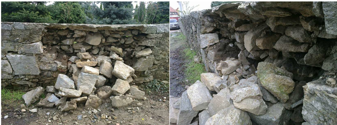
Figure 6: Free-standing two-layered wall in rural Poland, damaged through the separation of layers (source: own).
