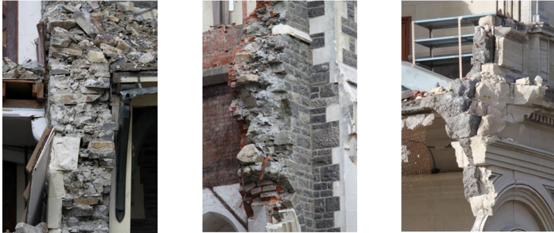
Figure 15: Stone masonry cross sections in New Zealand. From left to right: dressed stone in outer leaves and rubble fill, stone facing and brickwork backing, stone facing and concrete core (Source: NZSEE [98]).
