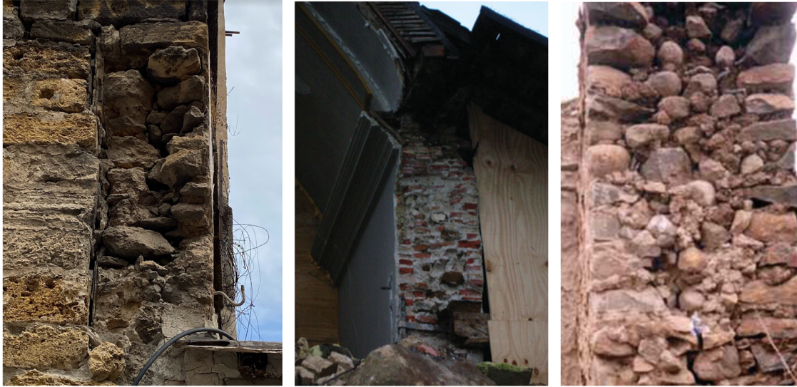
Figure 5: Exemplary three-layered masonry walls. Left: example from Palermo (Italy) – irregular stone cladding and very thin core consisting of small cobbles and pebbles (own source). In the center: brick masonry with regular cladding and core with high mortar ratio – Meldert-Lummen (Belgium). Right: uncoursed random rubble stone wall, stone cladding, and core made of cobbles in a matrix of mud mortar (Maharashtra, India) (source: own and previous studies [41,42]).
