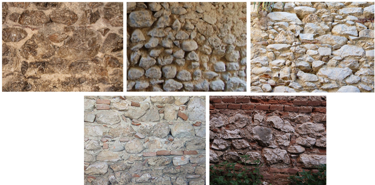
Figure 4: Example of masonry types in L'Aquila (Central Italy) (after Rovero et al. [40]).
