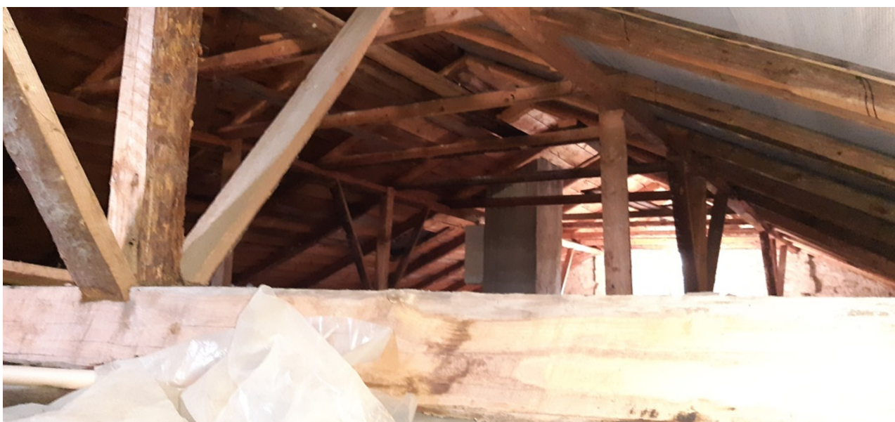
Figure 5: View of the roof structure.
