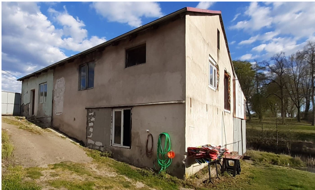
Figure 4: View of the north and west walls.
