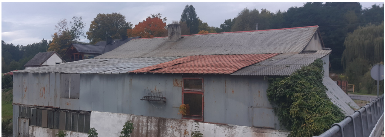
Figure 6: View of the building from the south.
