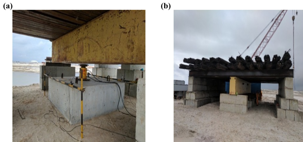
Figure 2: (a) Typical setup of footing load test (India and Nigeria). (b) Setup of footing load test (Dangote refinery site, Nigeria).
