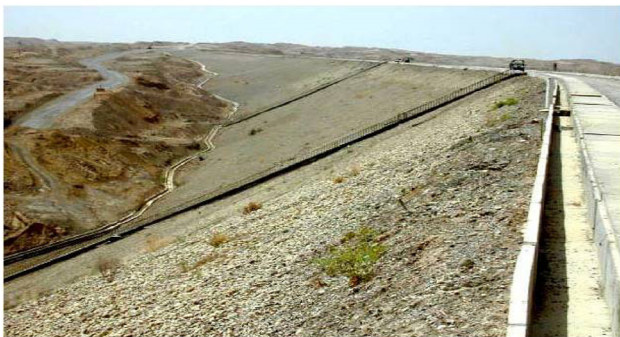
Figure 2: Al-Adhaim dam (Al-Labban, [30]).
