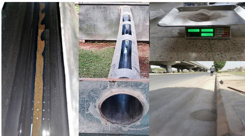
Figure 1: The sand collection and sediment occurrence on the bed of the pipe.
