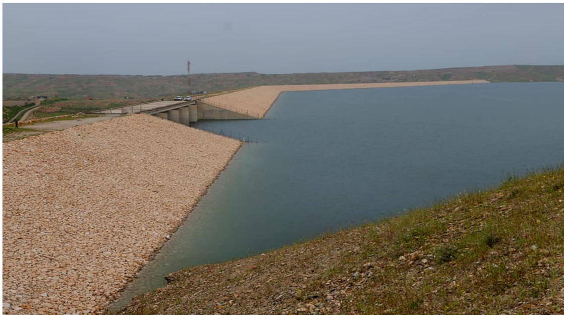
Figure 2: Khassa Chi dam currently.
