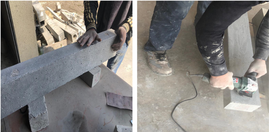
Figure 8: Configuration steps of the preparation surface RC beams to increase the adherence of BFRP by epoxy.
