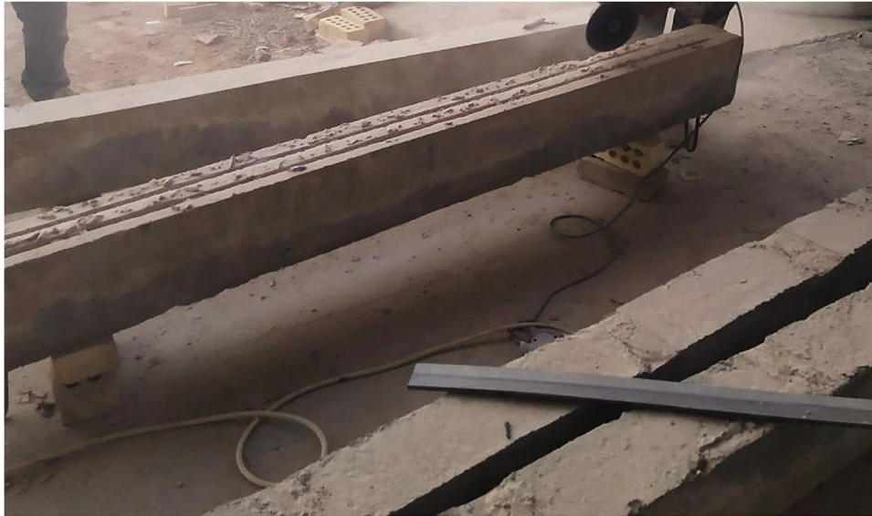
Figure 3: Cut off the grooves.
