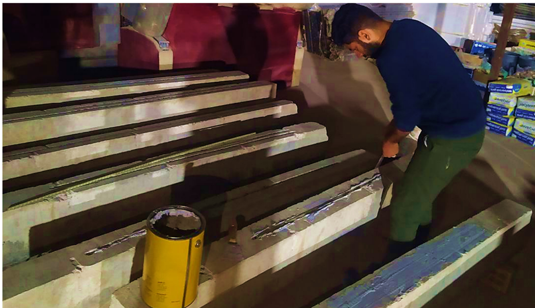
Figure 4: Application of NSM bars.
