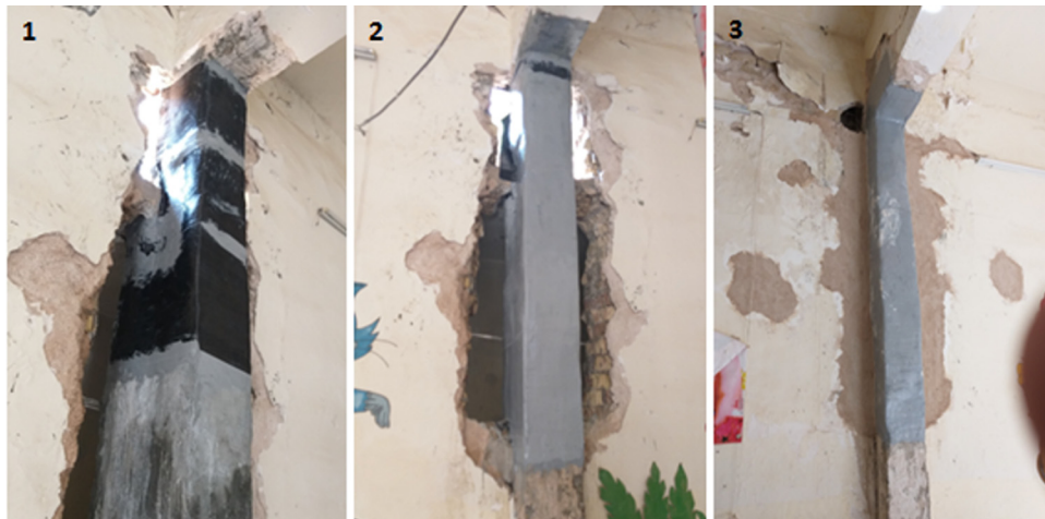
Figure 4: Wrapping columns by using CFRP sheet.
