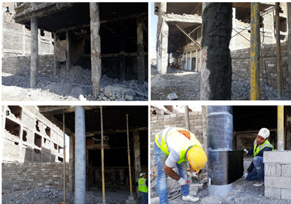
Figure 2: Steps involved in repairing and strengthening RC columns in Al-Mosul city.
