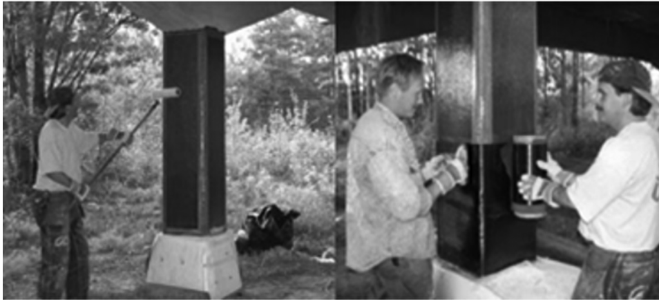
Figure 1: Strengthening of RC columns by FRP sheet in Sweden, photo by Täljsten [34].
