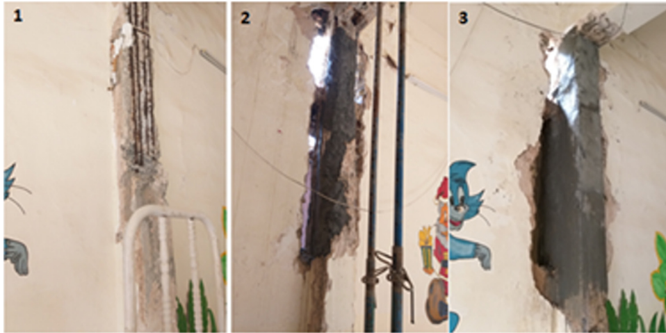
Figure 3: Cleaning and coating concrete surface.
