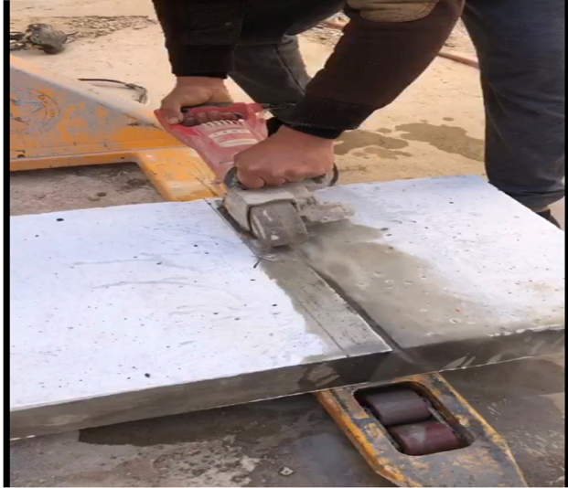
Figure 3: Making grooves.
