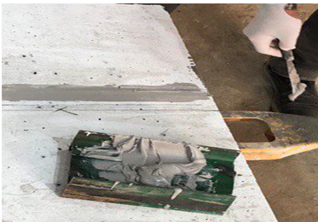
Figure 5: Mixing of epoxy paste.
