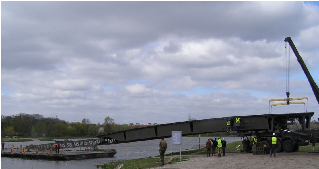
Figure 3: MS-40 bridge being placed on a floating support.
