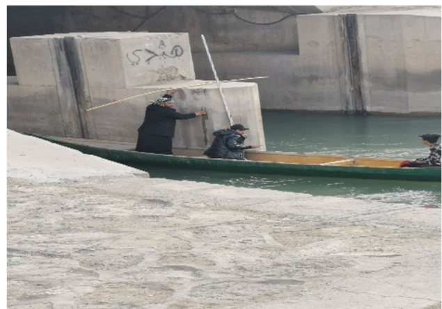
Figure 2: Survey work using level and the boat to survey the inside of the river.
