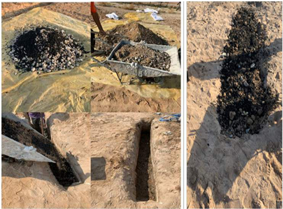
Figure 13: Trench filling stages.
