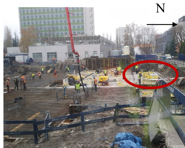
Figure 3: An image showing the construction site marking the shielding location during the concrete casting. Own source, 25.11.2019.
