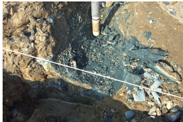
Figure 11: A view of BAT piezometer before installation into a cut-of wall.
