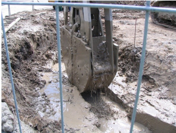
Figure 2: A view of cut-off wall construction.
