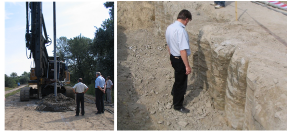
Figure 3: DSM technology.
