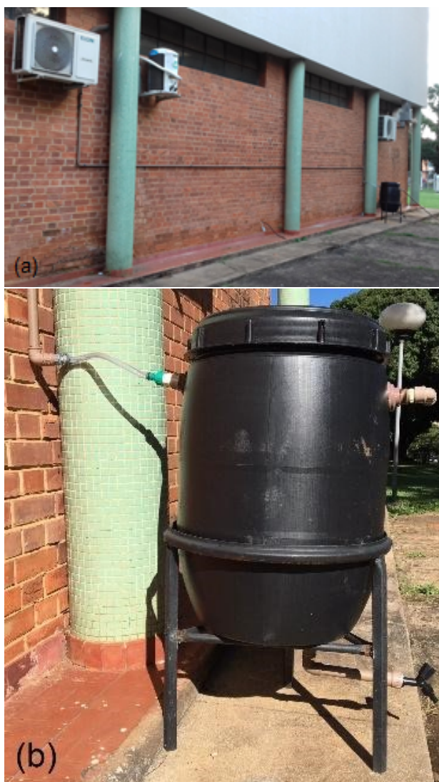
Figure 1: The water storage and collection system located outside the Laboratory of Water Analysis of the Federal University of Goiás (a), as well as the detail of the reservoir for the storage of collected water (b).
