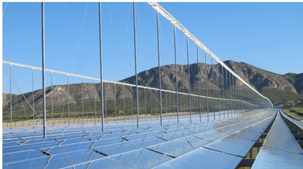
Figure 3: Linear Fresnel collector array, 1.4 MW PE1 plant in Murcia, Spain (Reve 2012).
