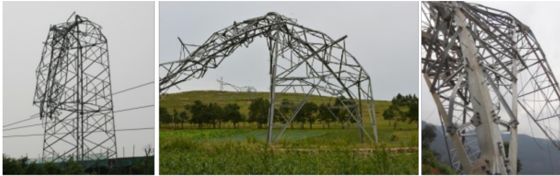
Figure 1: Collapse accidents of transmission tower
