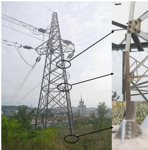
Figure 2: Actual angle joint of transmission tower
