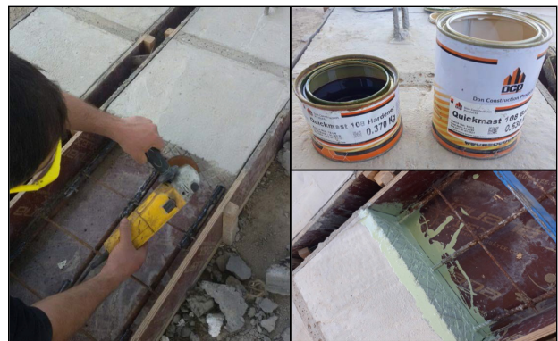
Figure 8: Preparing old concrete surface.
