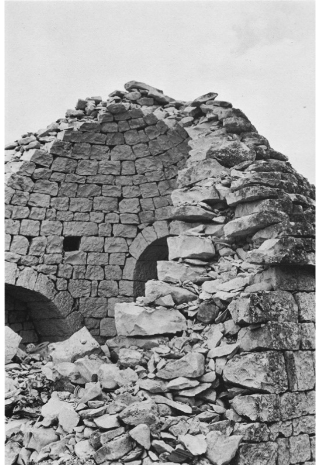
Figure 1: Example of the partial collapse of a Trullo vault [14].
