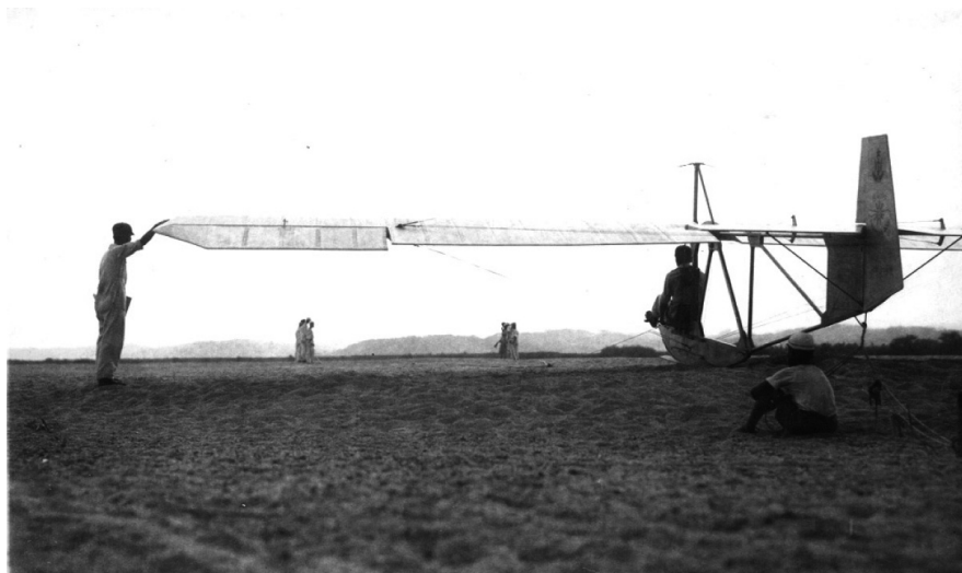
Figure 3: Low tech, high aims: A Monbushōgata Puraimarī glider shortly before takeoff. In the background the launching crew is preparing to stretch the two bungee cords that will catapult the glider into the air. The photo gives a sense of the rudimentary technology as well as the teamwork involved. Courtesy of Vintage Sailplane Historical Association, Fukuoka.
