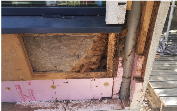
Figure 5: Facade opening during the restoration of water damage.
