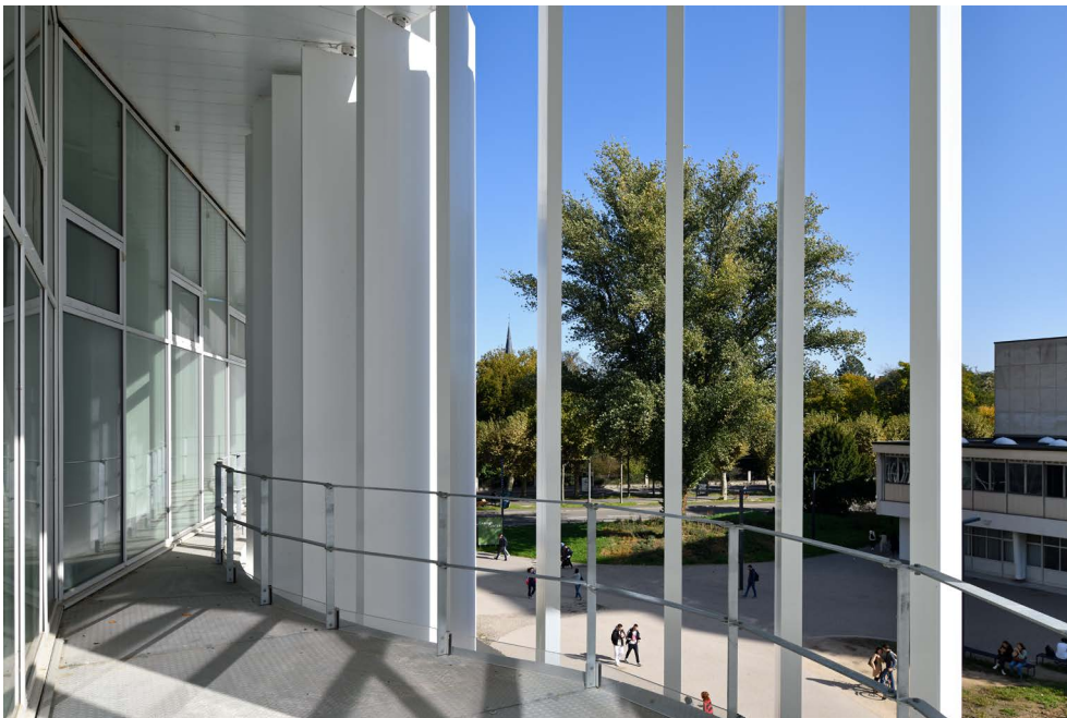
Abb. 8: The vertical strips help to maintain the building's thermal environment and light levels (photo: C. Bourgeois)
