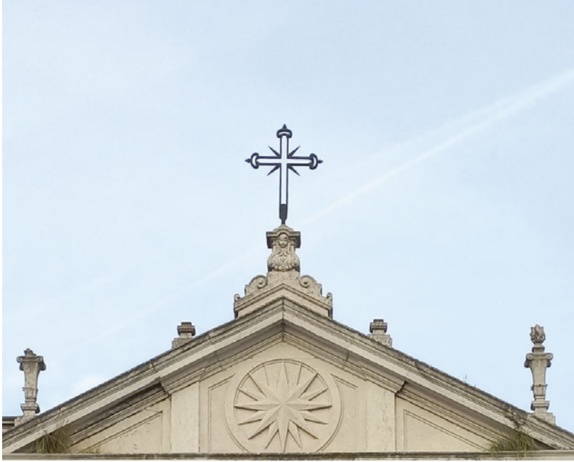
Figure 7.2. Top of the façade of the church of Our Lady of Needs (Nossa Senhora das Necessidades) in Lisbon. The baroque budded cross at the top, with the diagonal rays, seems to visually replicate the sixteen rhumbs of the wind rose below. This church was the home of the Lisbon Oratorian Fathers, who in later times, for about a century, taught mathematics, astronomy, and other disciplines to the Portuguese navigators. 54 The harmony between the cross, representing meta-physical and theological doctrines, and the technoscientific division of space, represented by the wind rose, is in perfect agreement with the “vertical” vision of world-crafting laid out in Timaeus and verified at every turn throughout the Middle Ages. For a detailed study of this question, down to the thirteenth century, see Acevedo, Alphanumeric Cosmology from Greek into Arabic .
