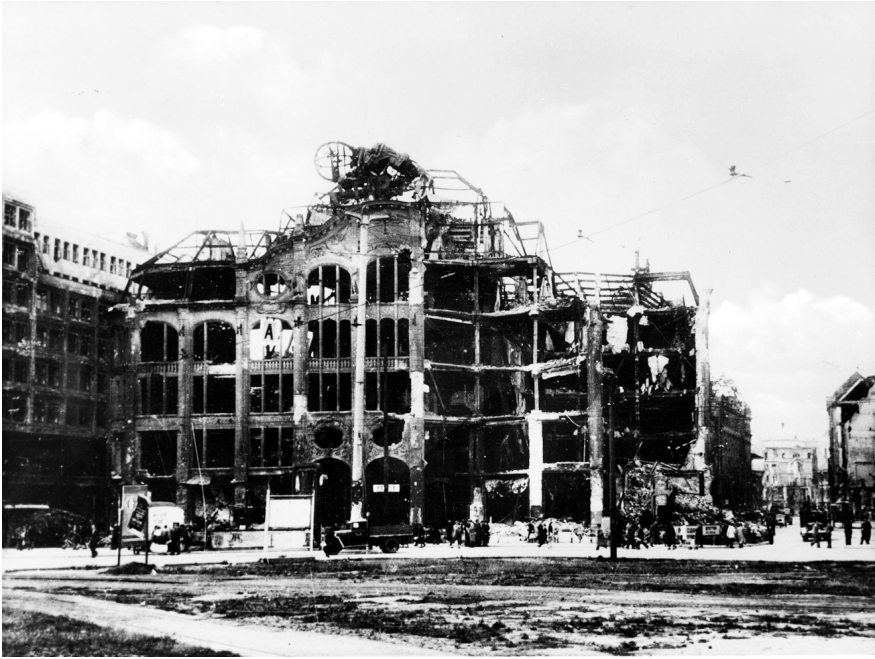
Fig. 29: The war-torn Hertie department store on Berlin Alexanderplatz, around 1945.
