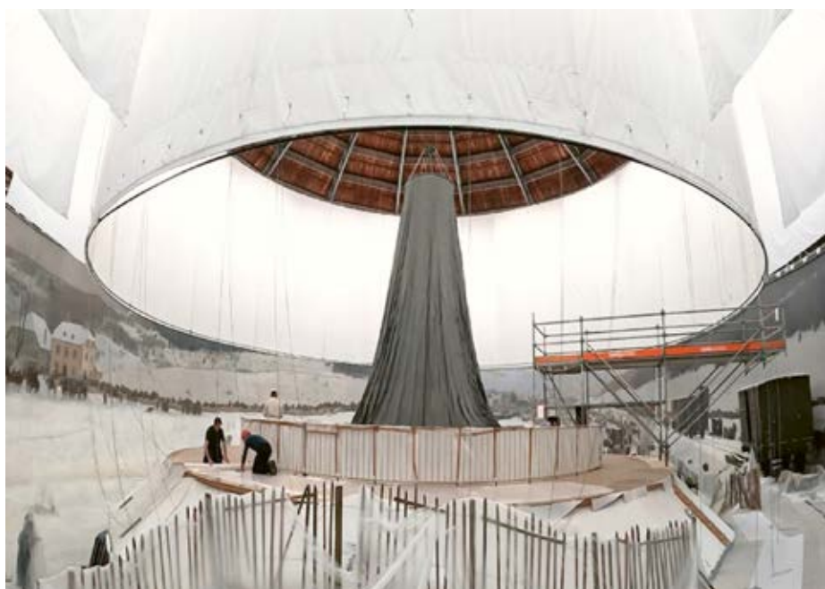
Fig. 15: Parts of the faux terrain and platform protected with plastic film. In the center, the new canopy being lifted into the cupola, 2024. Image, Bourbaki Panorama Foundation.
