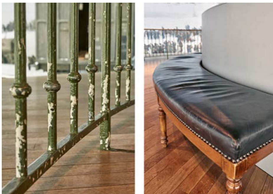
Fig. 7: Signs of wear and tear on the historic components of the visitor platform, 2023. Images, Bourbaki Panorama Foundation, Lucerne.
