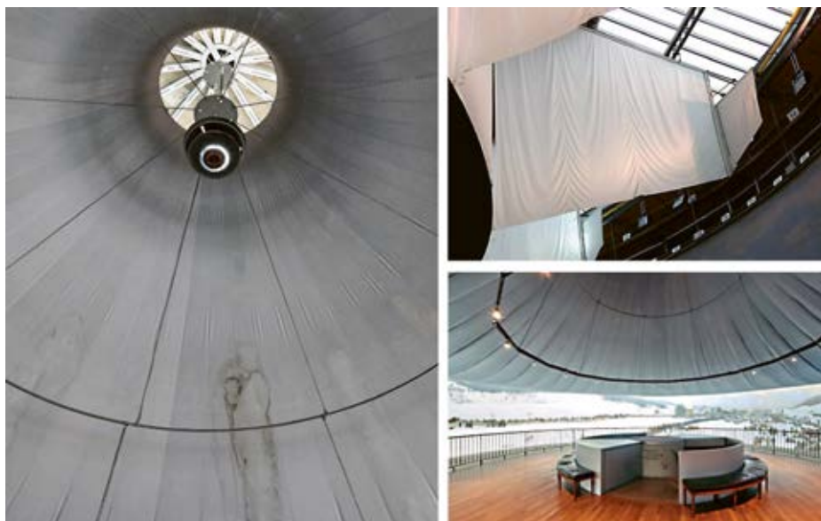
Fig. 6: Stains and rainwater rings on the canopy, and sagging of the velum fabric due to ageing, 2023. Images, Bourbaki Panorama Foundation, Lucerne.
