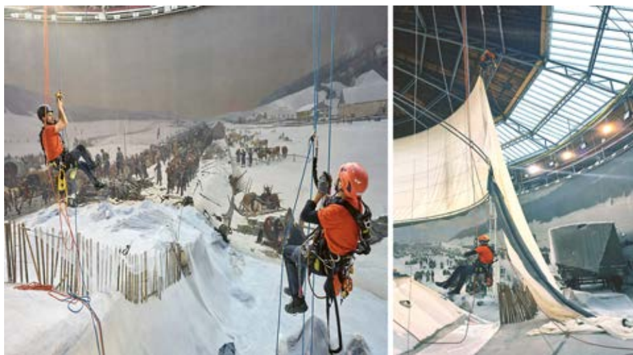
Fig. 14: Industrial climbers dismantling the old canopy, 2024. Images, Bourbaki Panorama Foundation.
