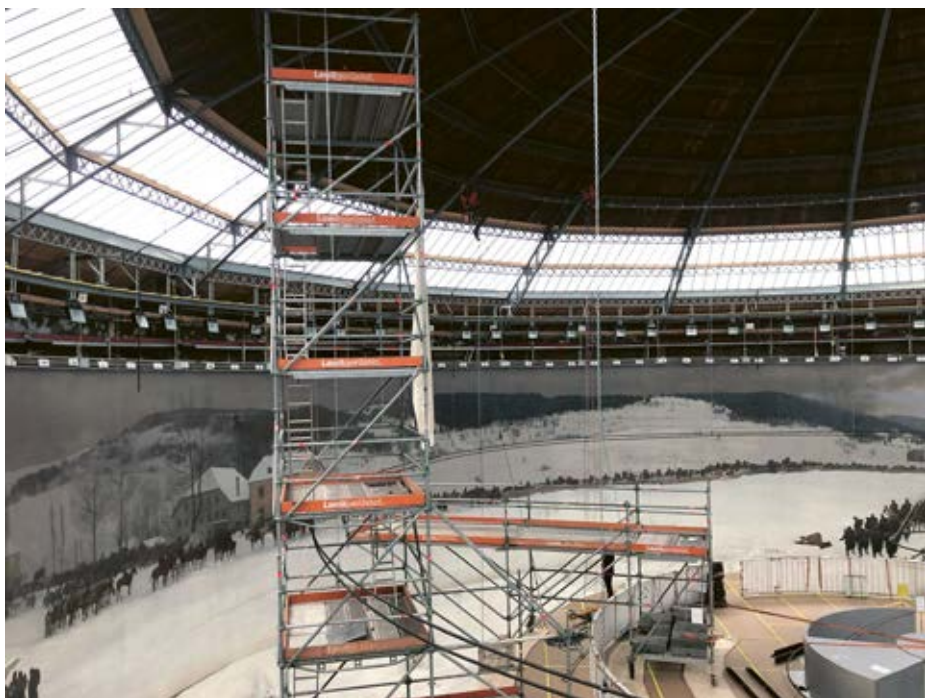
Fig. 13: Scaffolding for the assembly of the canopy, velum and the sun sails, 2024. Image, Bourbaki Panorama Foundation, Lucerne.
