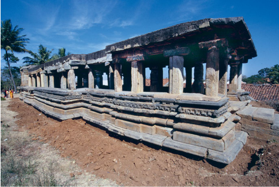
Plate 5.4: The prominent moulded plinth, adhiṣṭhāna , of the large double temple at Kambadhalli. The second shrine, at the eastern end (front of photo where the steps are), was destroyed.
