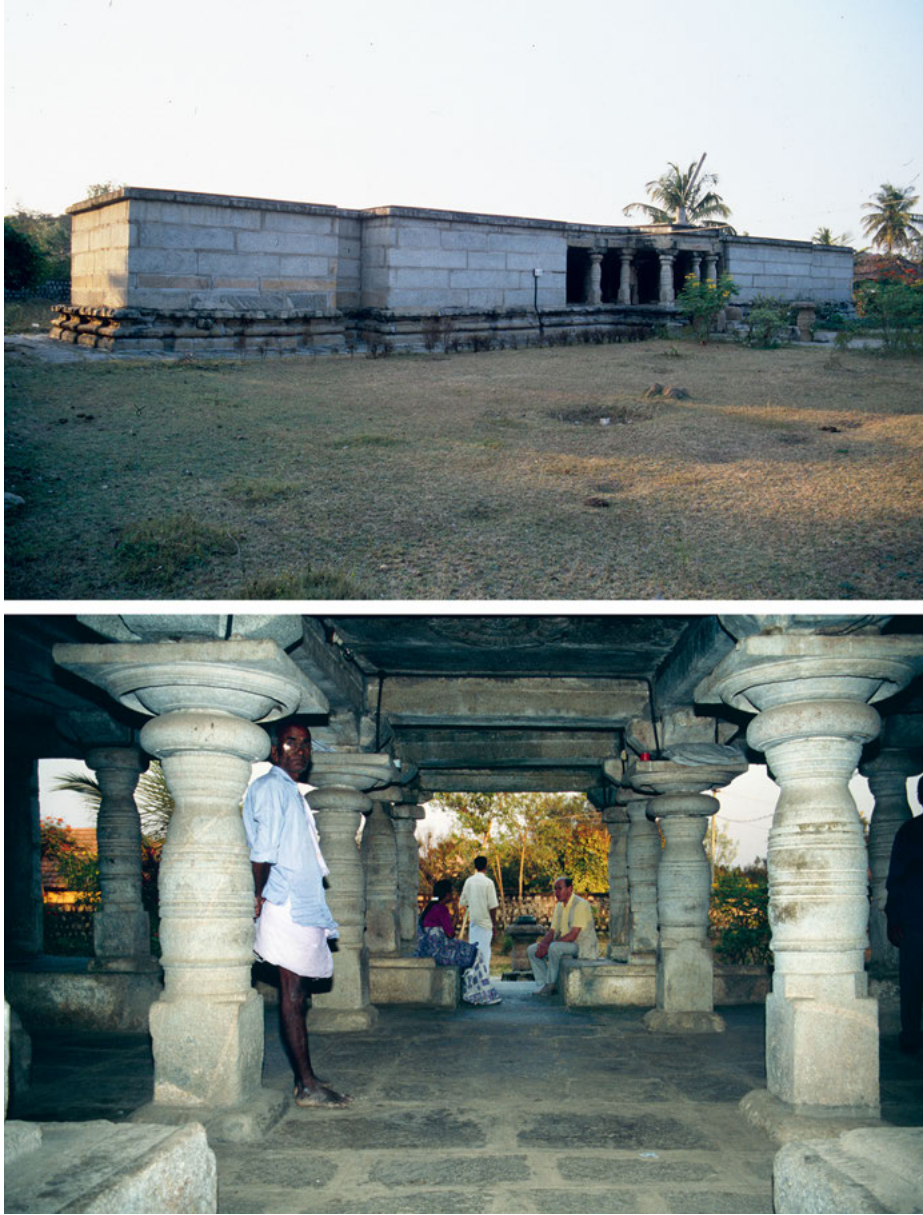
Plate 5.34: The late-Hoysala Ādinātha Trikūṭa Basadi at Chikka Hanasoge was built on a much larger plan but its lathe-turned pillars are shorter and the ceilings simpler than at other sites of the period.
