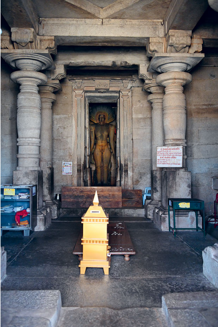
Plate 5.30: View towards the sanctum inside the early twelfth-century Antarāla Pārśvanātha Basadi on Candragiri, which has tall lathe-turned pillars inside its navaraṅgamaṇḍapa .
