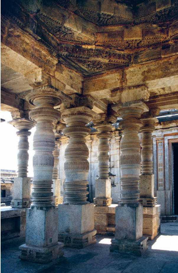
Plate 5.22: In the detached open hall of the Pārśvanātha Temple at Halebidu are fourteen highly polished lathe-turned stone pillars, which are typical of later Hoysala basadis .
