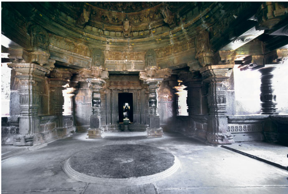
Plate 5.20: The late twelfth or early thirteenth-century Kamala Basadi at Belgaum has an open pillared hall, navarāṅgaṃḍapa , with lathe-turned pillars and an elaborate domical lotus ceiling (below).
