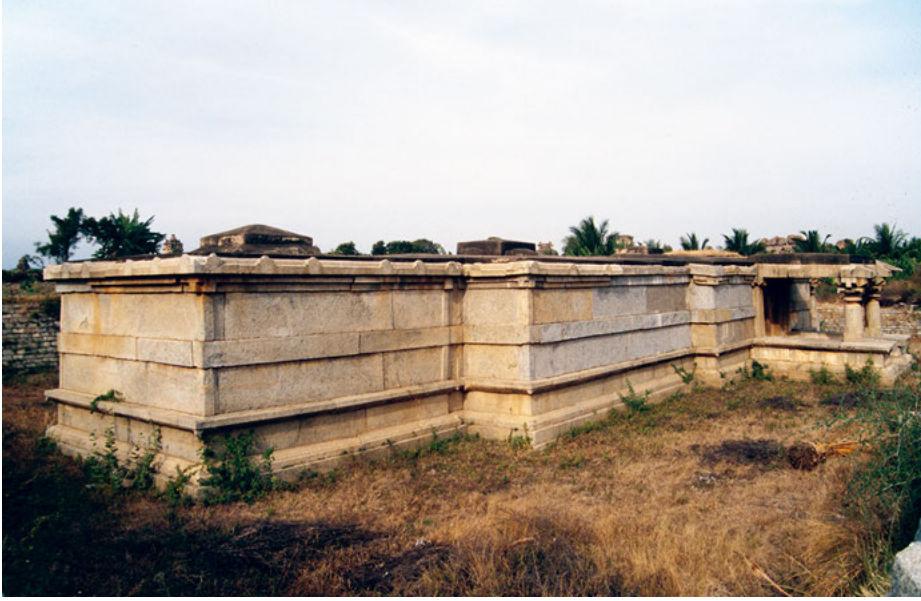
Plate 2.7: Rear view of the Pārśvanātha Temple, located close to the elephant stables inside the royal centre at Hampi.
