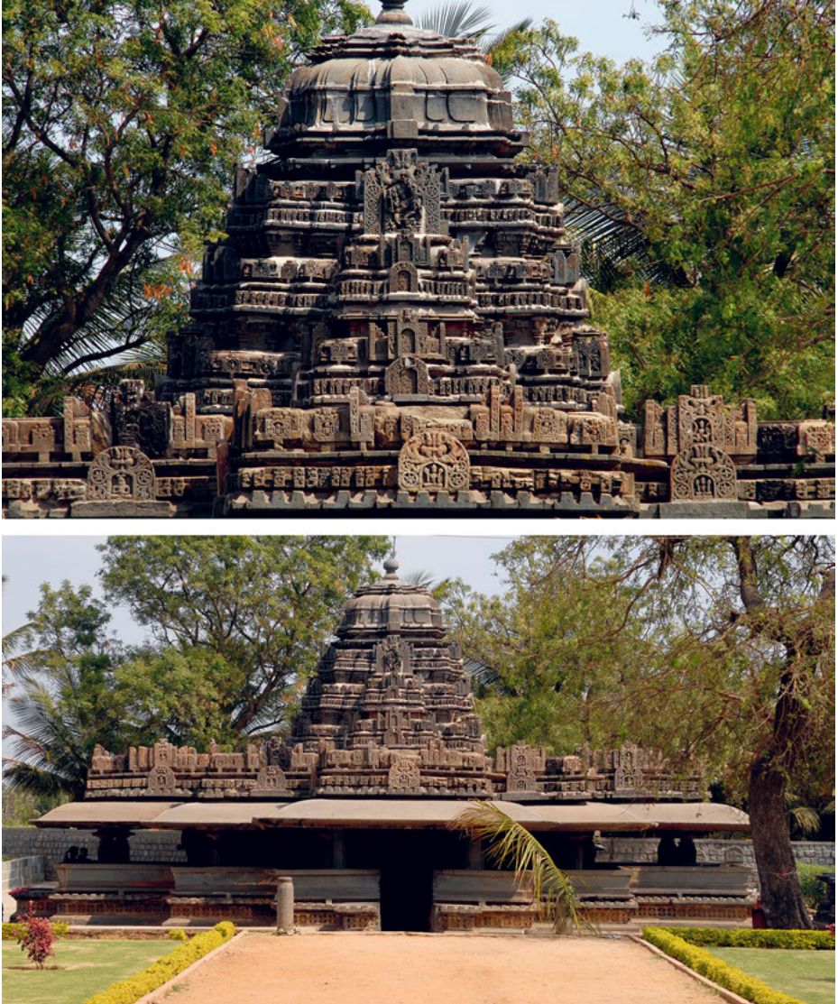
Plate 1.36: The former Digambara Jaina Mallinātha Temple at Haveri was converted by Viraśaivas, who named it the Vīrabhadreśvara Temple and removed most Jaina statuary from its roof.
