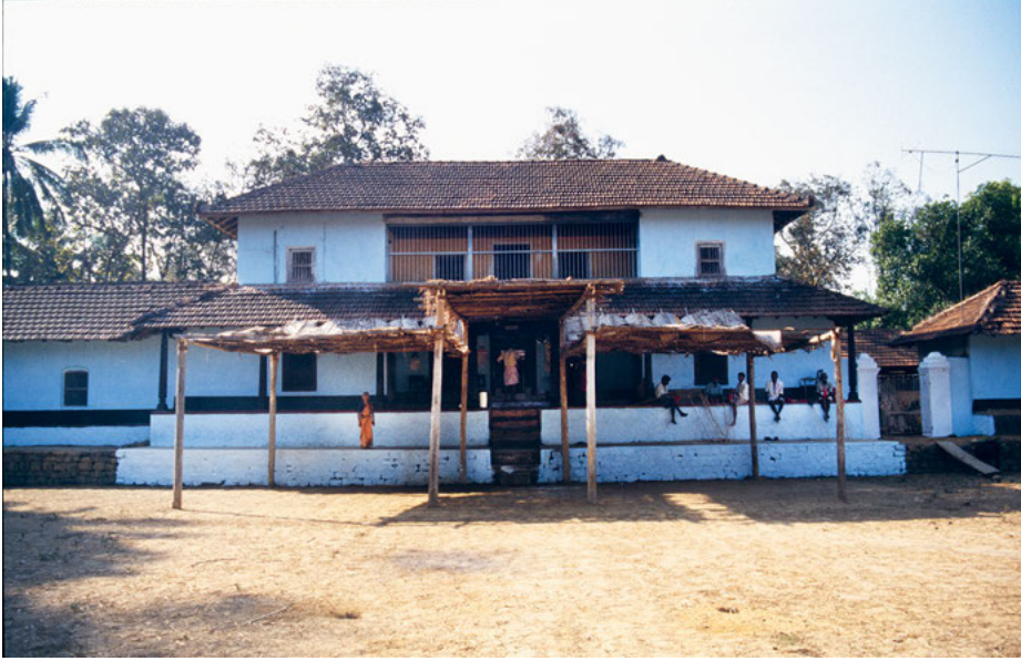
Plate 1.50: Entrance to the ancient Jaina matha at Varanga, displaying the typical sloping red tiled roofs, characteristic of the architecture along the coastal line of Karnataka, which has adapted to strong rains.
