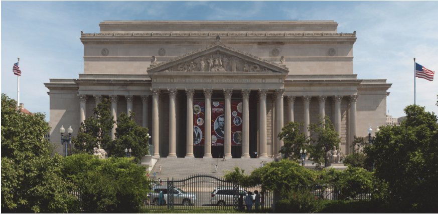
Fig. 21: National Archives Building, Washington DC, photo: David Samuel; CC BY-SA 3.0, via Wikimedia Commons: < https://commons.wikimedia.org/wiki/File:US_National_Archives_Building.jpg > (accessed on 5 December 2024).
