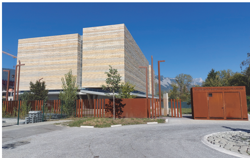
Fig. 19: Archives of the department of Isère, France, photo: Binnette; CC BY-SA 4.0, via Wikimedia Commons: < https://commons.wikimedia.org/wiki/File:Archives_d%C3%A9partementales_de_l%27Is%C3%A8re.jpg > (accessed on 5 December 2024).
