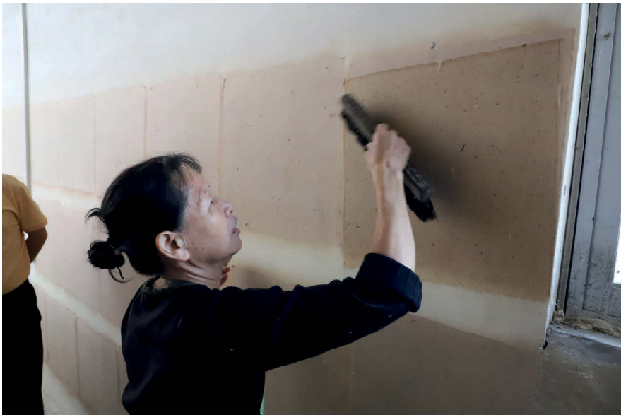
Fig. 15: Pasting the paper sheets on the wall for drying
