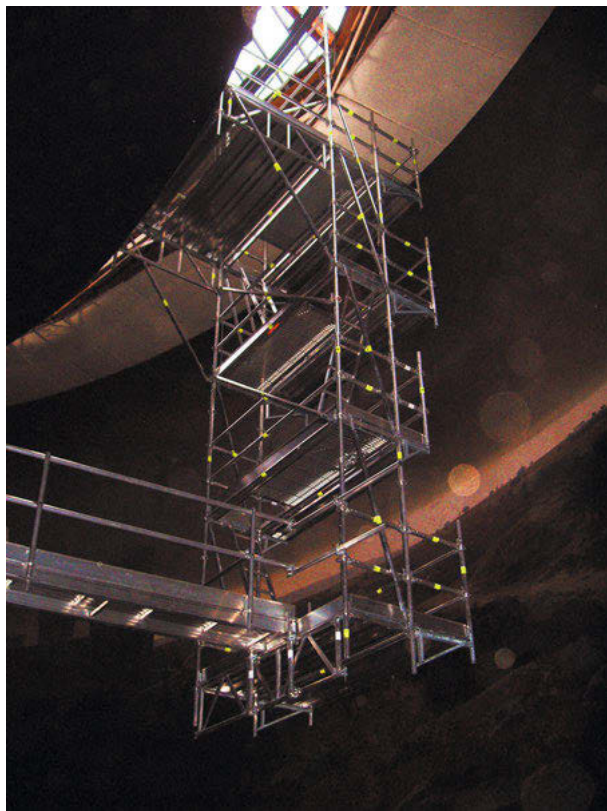
Fig. 4: Suspending light-weight scaffolding. Image, the author.
