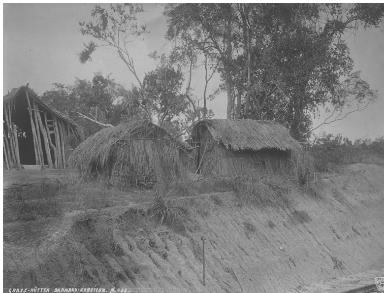
Figure 4: English: “Grass huts of railway workers, no. 458”.
