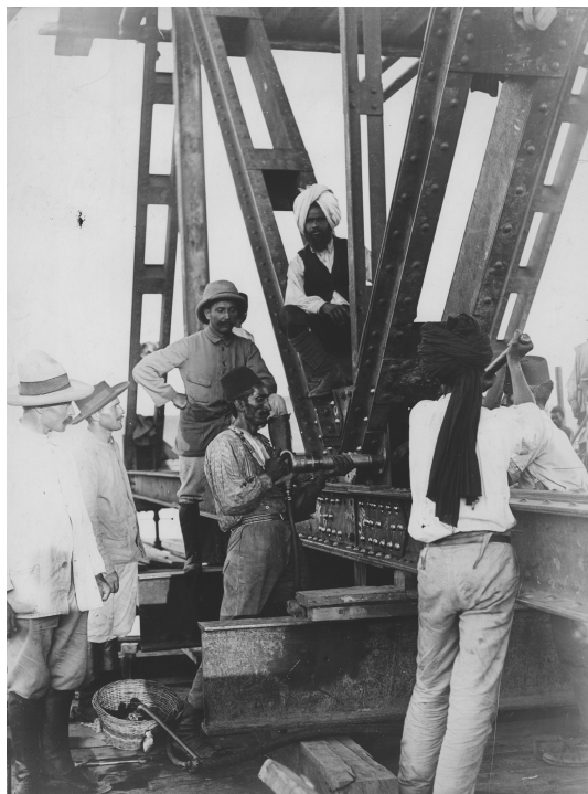
Figure 2: Indian craftsmen riveting bridge parts using modern machinery at the Malagarassi-Bridge 1912–13.
