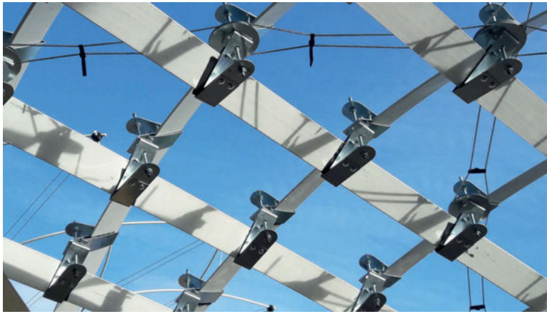
Fig. 9: The standard nodes developed in this study and bracing system. Laths cross-section: 100 \times 8 mm.
