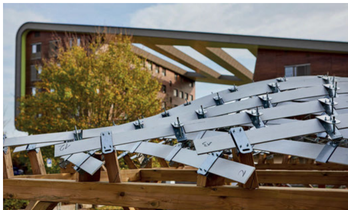
Fig. 4: The pseudo-geodesic pavilion, made of 100 mm GFRP lath at 60^\circ with a unique Z-connector. (Picture: Charlene Yves)
